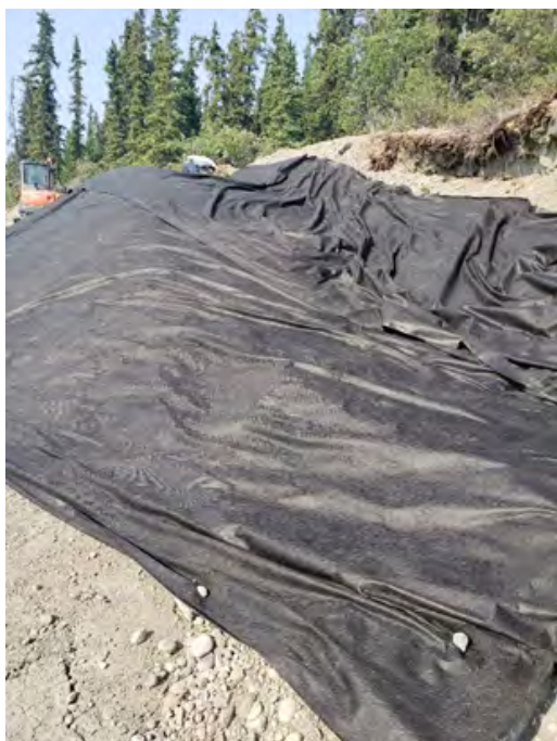
Figure 10: Technical Fabric covering the sand and gravel
