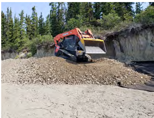
Figure 5: Access ramp development over technical fabric alongside the bank
