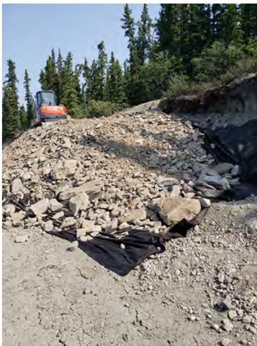
Figure 11: Angular rock to cover the entire mound
