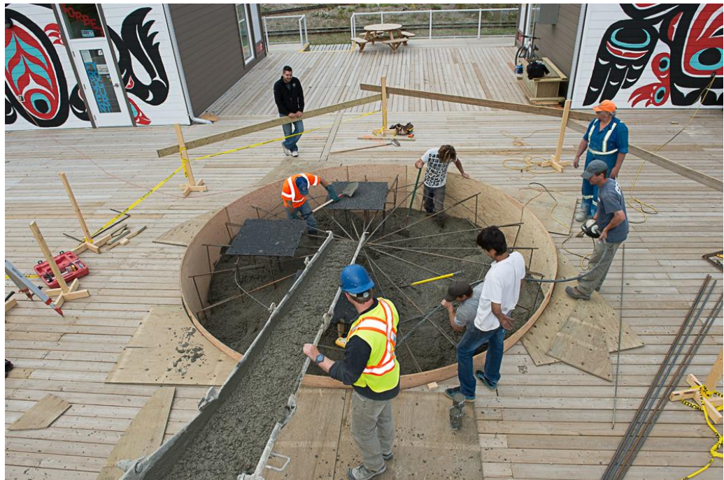
Preparing the massive foundation for the pole
